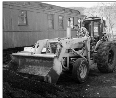
Denny Haefele spreads donated recycled asphalt on the north side of the Rico and RGS 20. – Photo © Bob Tully.
